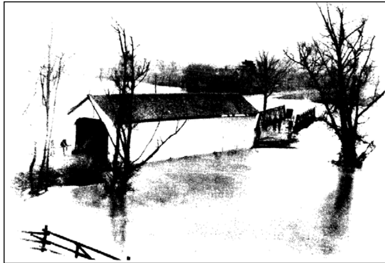
Figure 1. March 25, 1913 - Covered Bridge over Rocky River on Granger Road (Looking east)
